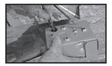
Drill a 1<sup>3</sup>/<sub>4</sub> inch hole and feed the conduit through the hole.
